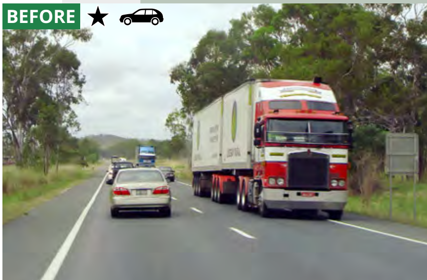
The “Bruce Highway” in Australia before and after being upgraded to improve safety.
